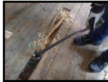
Breaking up wooden floors
